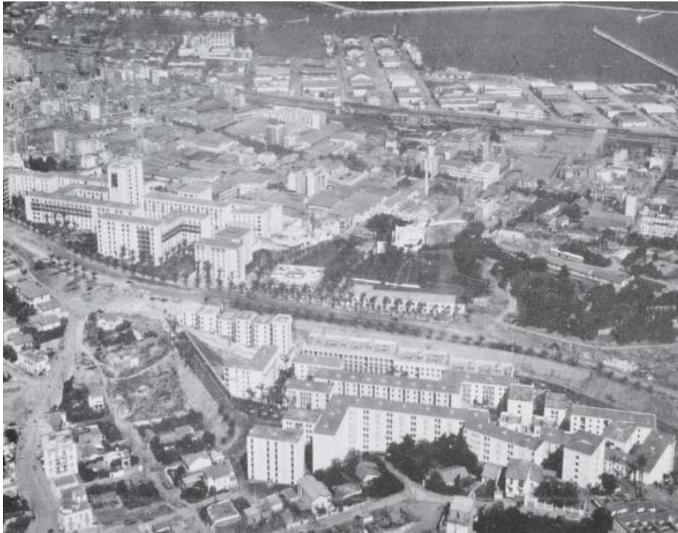
Figure 2. Cité Diar El Mahçoul, high comfort (background) and medium comfort (foreground). Spring : Revue chantiers, revue illustrée de la construction en Africain du Nord, N°23, Alger, 1956.
