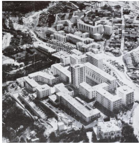
Figure 3. View of the two districts: high comfort (foreground) and medium comfort (background), Cité Diar El Mahçoul. Spring : Revue chantiers, revue illustrée de la construction en Africain du Nord , N°23, Alger, 1956
